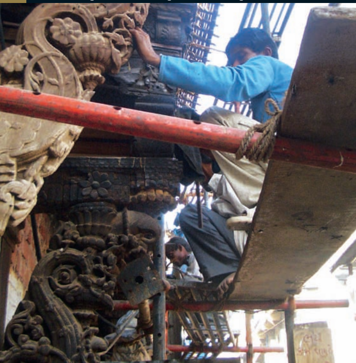
Restoring the Jalali mosque in Ahmedabad (India).
