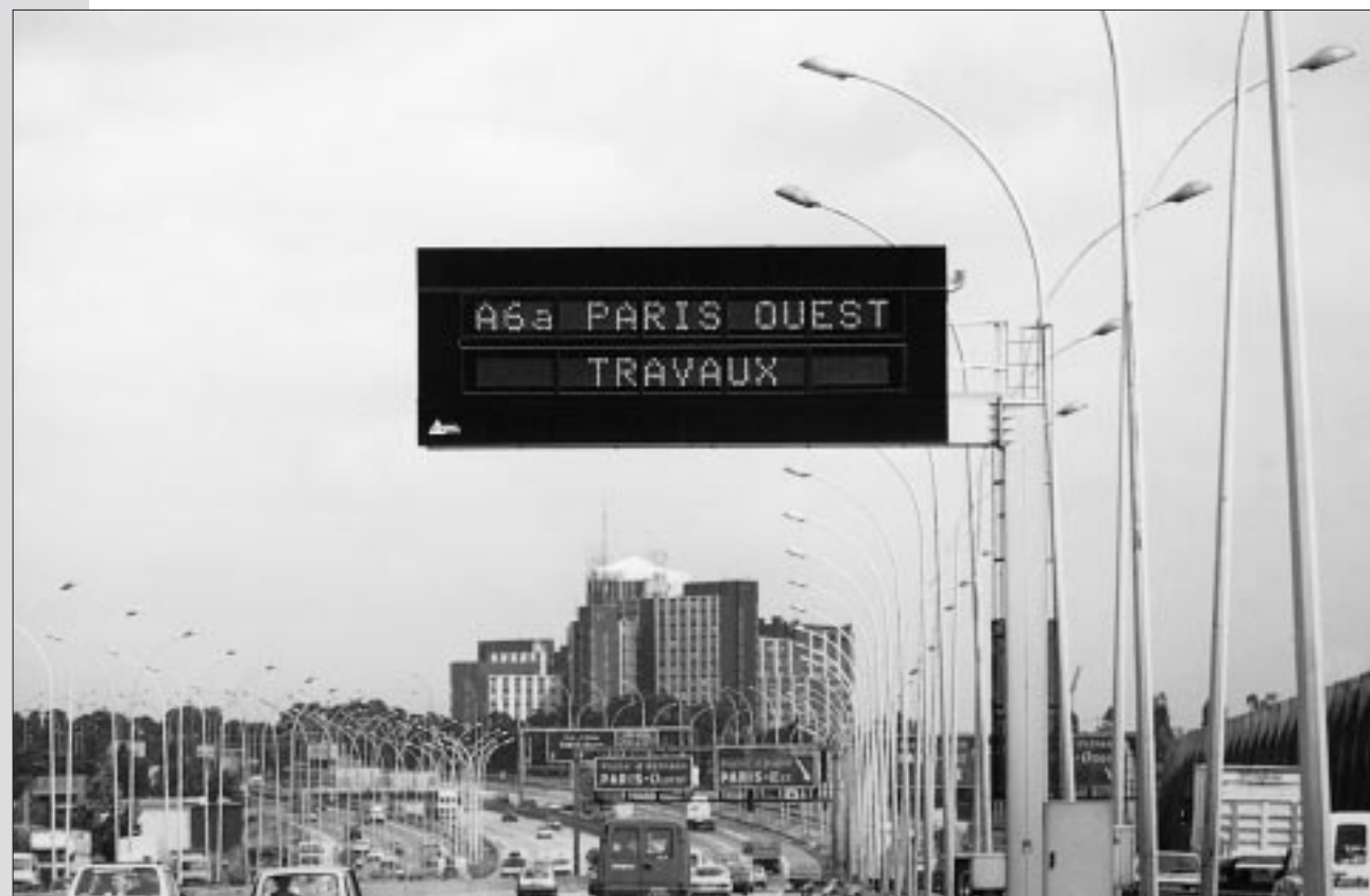
The constantly updated SIRIUS-system variable message signs aim to inform rather than to advise.
