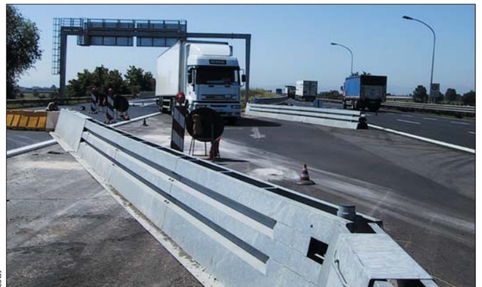
Median bypass (ITCP) on the A21 motorway (Italy).
