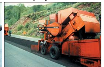
Cold mix recycling.
